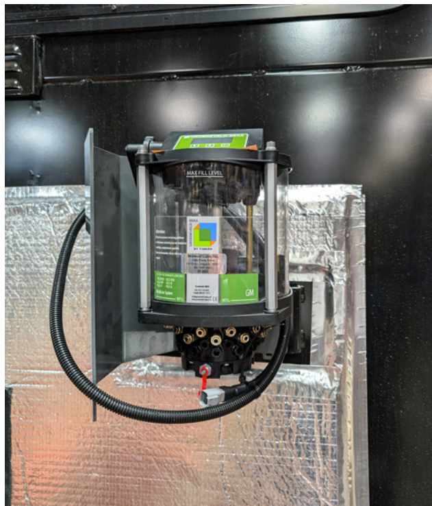
Fig. 35: Auto Lube Motor and Dispenser
