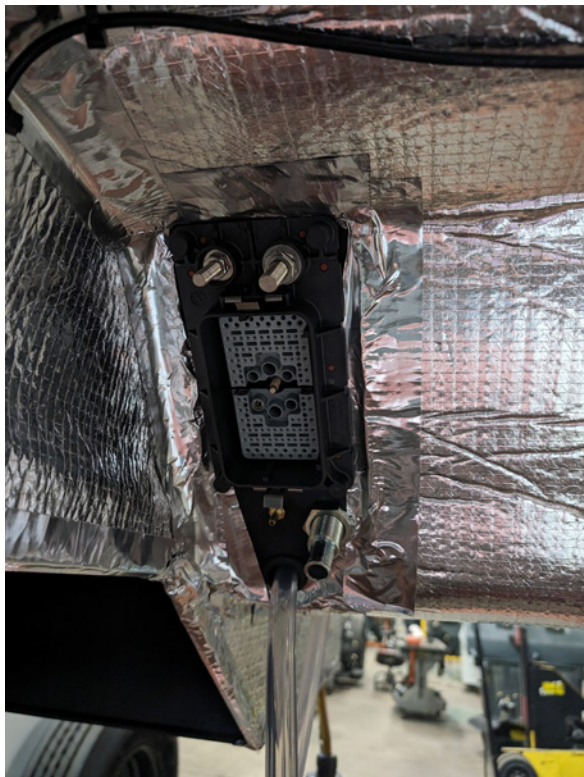
Fig. 20: External Ground Stud (Underneath Cab)
